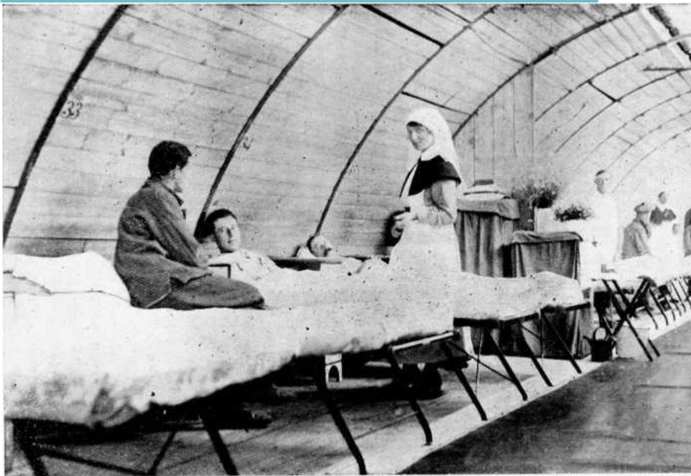
"HEAVEN"! A HUT IN FRANCE.
